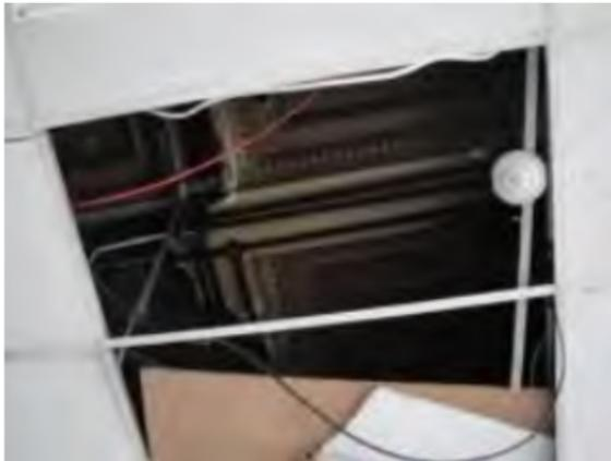
Evidence of damaged moulded plaster ceiling of former Banking Chamber
