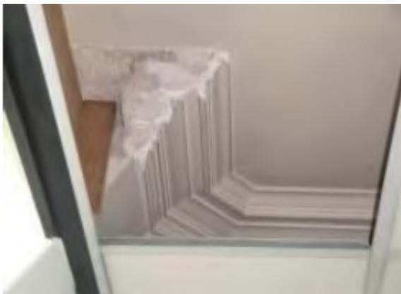
Typical cornice detail and damage incurred by alterations to windows/ installation of suspended ceilings.
