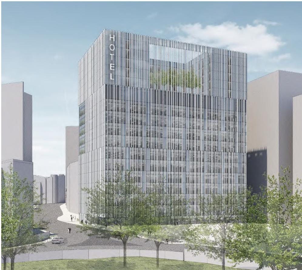
A veil comprised of Polyester Powder Coated fins would surround the building to provide a constant façade without revealing the changes in the facade between the
