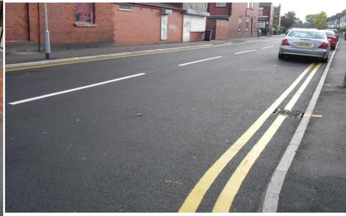
**Condition 2 “Signs of surface wear”** = Good condition – may comprise modular construction with elements of different colour/age/material, Faded bituminous materials (especially coloured bituminous), Graffiti or Spray paint etc. – **BLUE**
