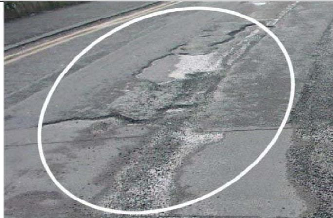
**Condition 5 “Structurally impaired”** = As grade 4 together with major signs of defects to structural layers or compromised sub base visible – **RED**
