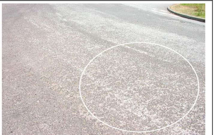
**Condition 3 “Mid-life”** = Signs of defects i.e. cracking, fretting, potholes, subsidence etc – all defects below intervention levels. – **GREEN**
