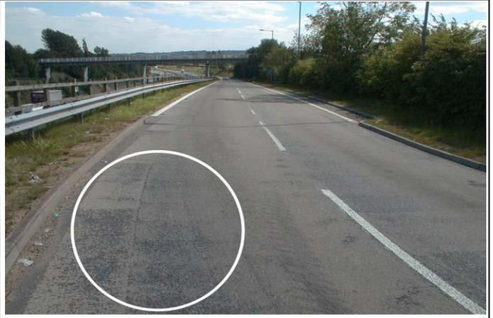
**Condition 4 “Functionally impaired”** = Signs of defects i.e. cracking, fretting, potholes, subsidence all defects above intervention levels – **AMBER**
