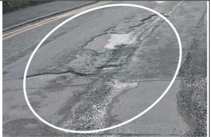
**Condition 5 “Structurally impaired”** = As grade 4 together with major signs of defects to structural layers or compromised sub base visible – **RED**
