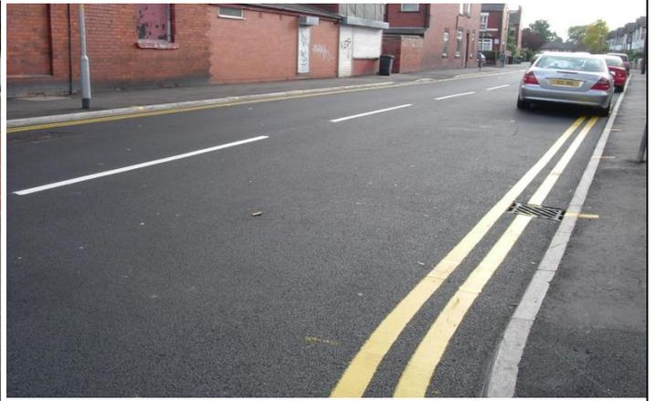
**Condition 2 “Signs of surface wear”** = Good condition – may comprise modular construction with elements of different colour/age/material, Faded bituminous materials (especially coloured bituminous), Graffiti or Spray paint etc. – **BLUE**
