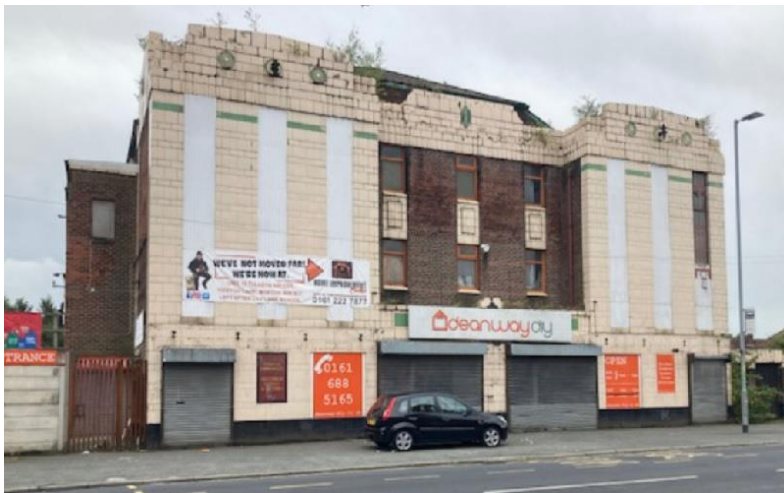
Existing building when viewed from Kenyon Lane
