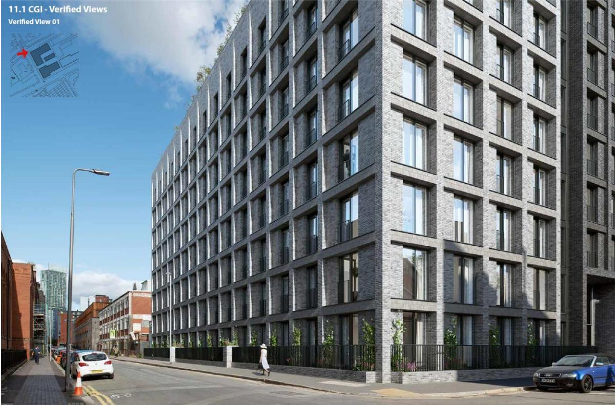
The taller section of Block B, at the junction of Chester Road and Hulme Hall Road, would be clad in dark grey metal with black window frames and balustrading to the balconies. It would strong grid lines with vertical and horizontal profiled metal fins creating a sharp geometric grid pattern.
