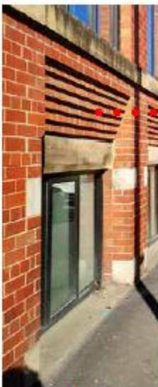
Brick detailing to openings - Britannia Mill
