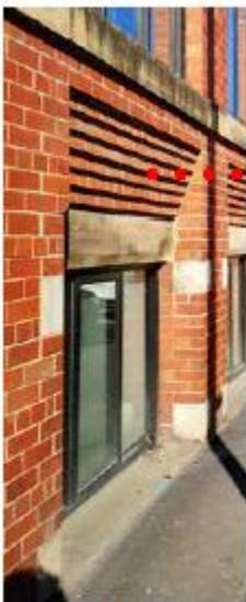
Brick detailing to openings - Britannia Mill
