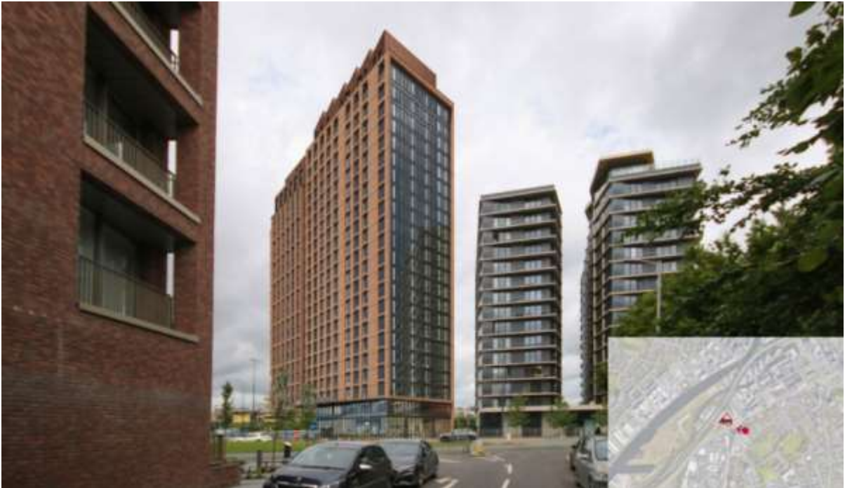
View From Princess Street Looking West
