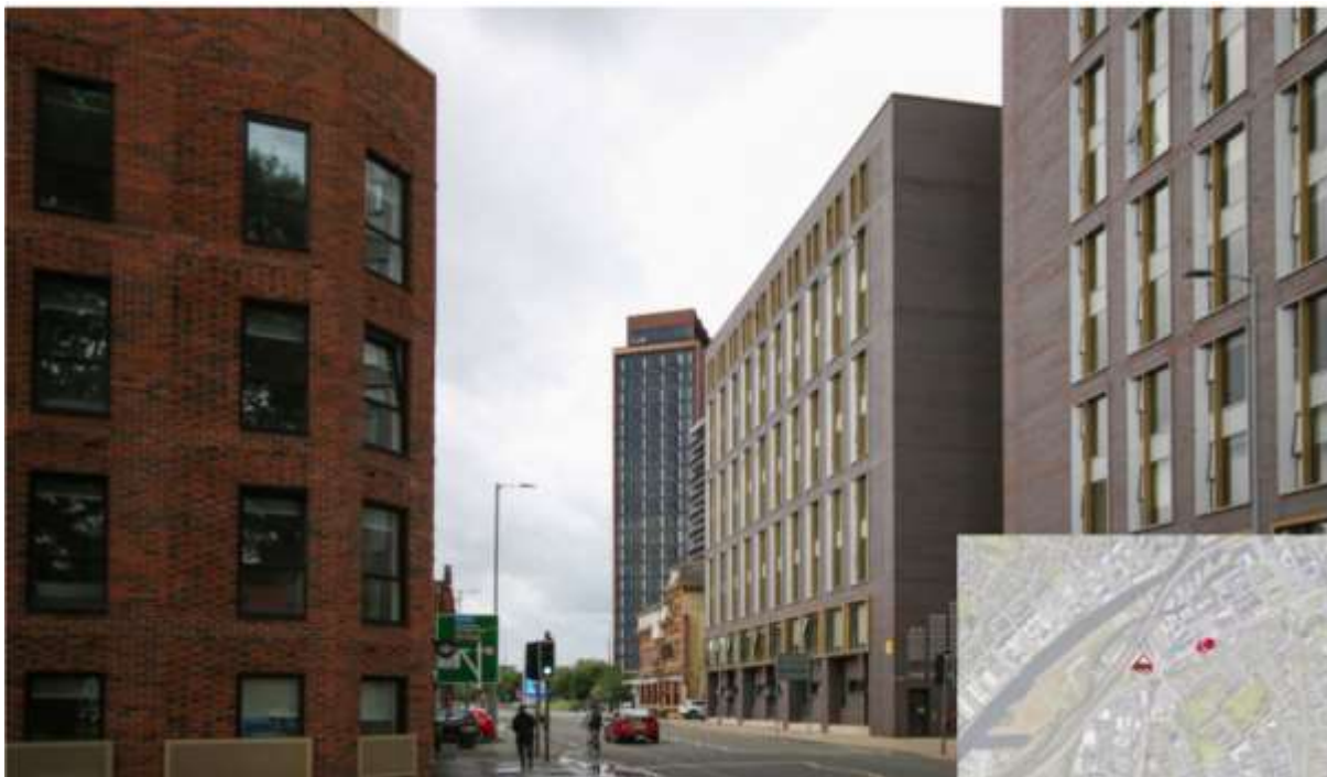
View From A56 Looking South-West
