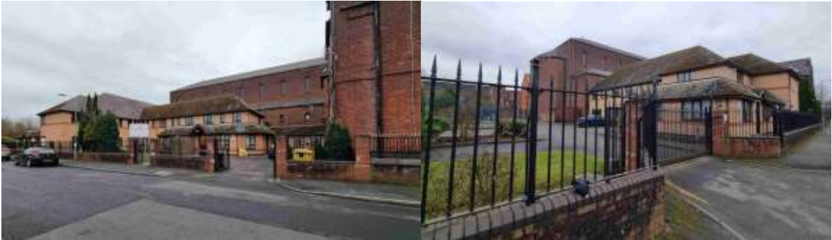
Photographs of front and rear of site as seen from Nobby Stiles Drive
