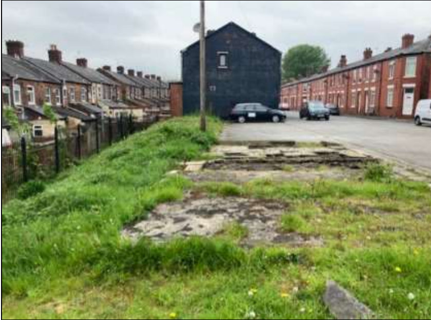
View looking towards the gable of the existing end terraced property on Clevedon Street.
