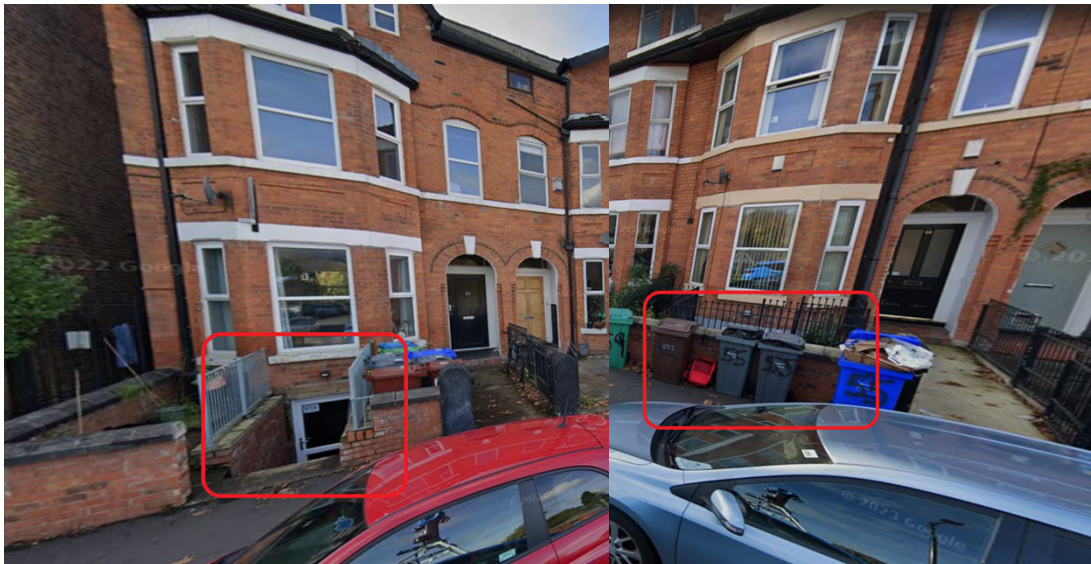
Door to basement of number 51 Albany Road (to the left) and basement window to 55 Albany Road as referenced in the assessment
