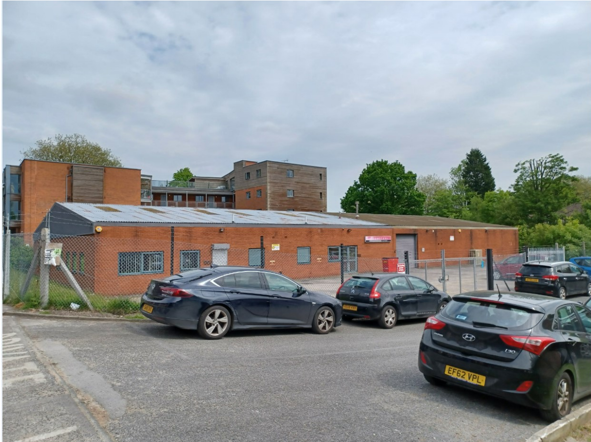
Application site together with single storey building to be demolished and Quadrangle residential apartment in the background, the access road into Albany Road Trading Estate is in the foreground
