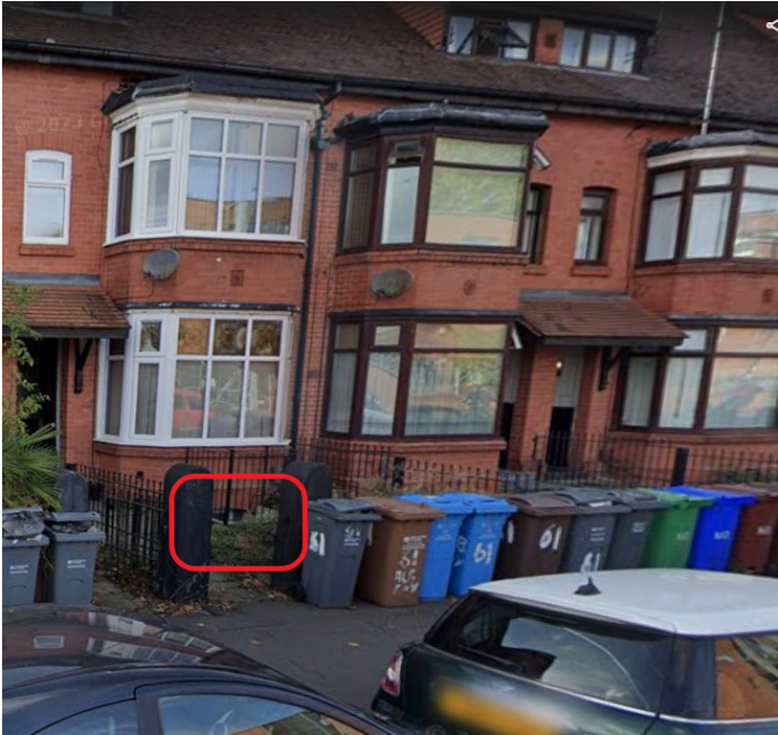
61 Albany Road – position of basement window is edged red
