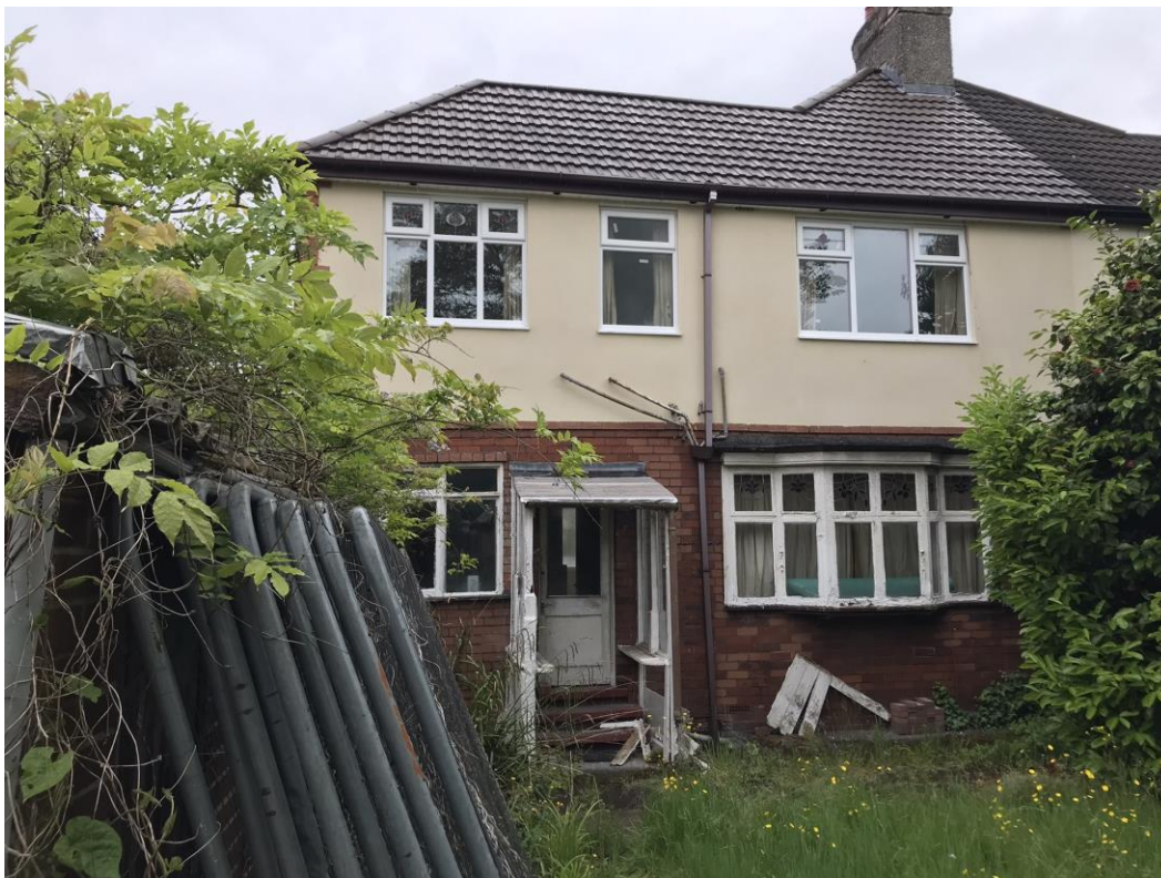
Existing rear elevation of the property
