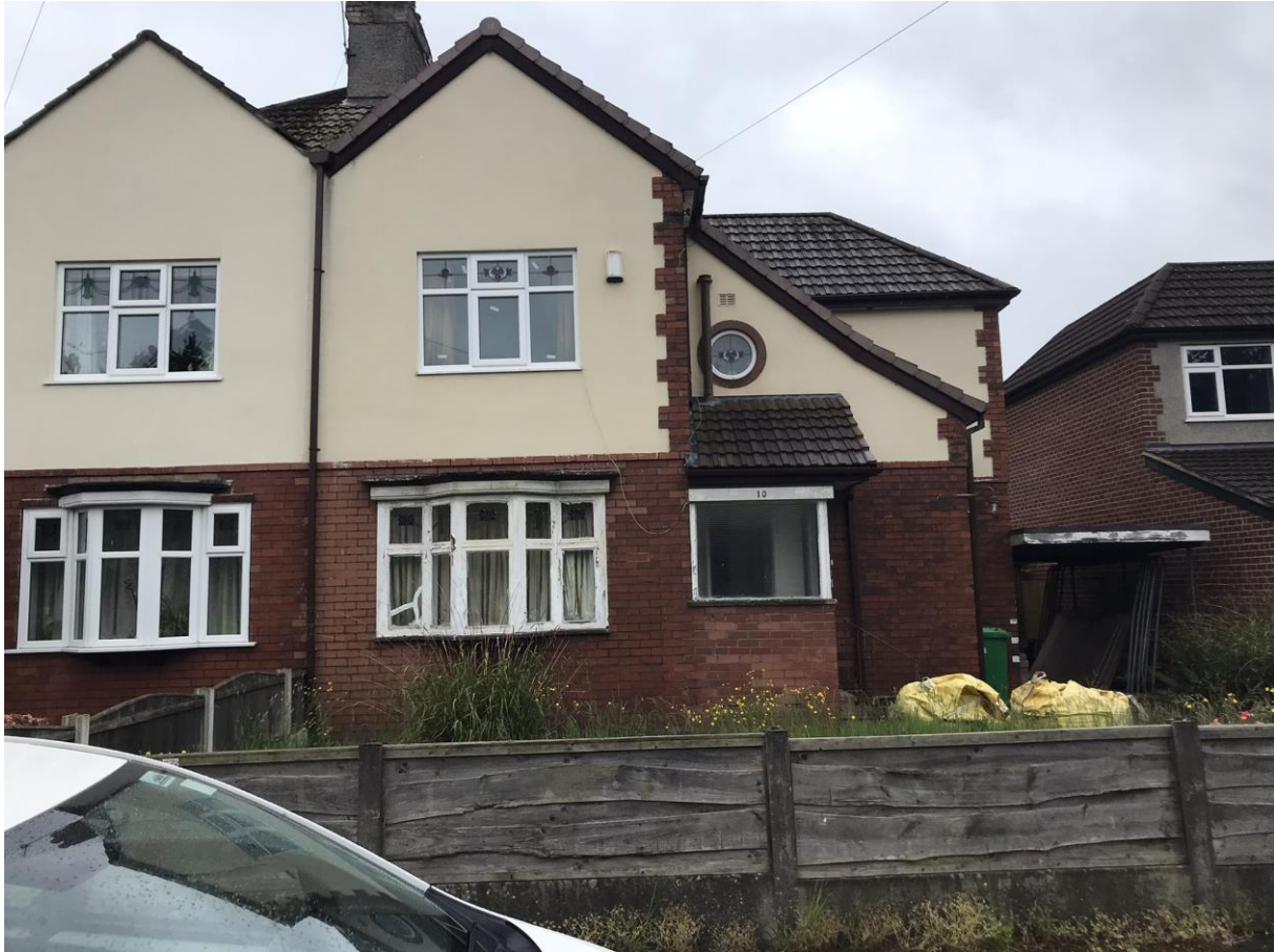
Host property's relationship with no.8 Ruabon Road's western elevation
