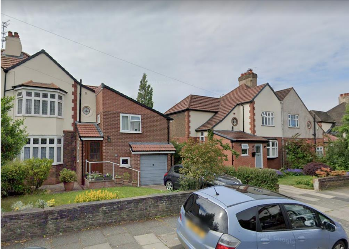
Example of no.16 Ruabon Road's single storey front extension and no. 18 Ruabon Road's two storey front extension
