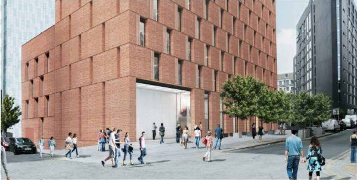
Main entrance off Hulme Street including patter brick work to Great Marlborough Street
