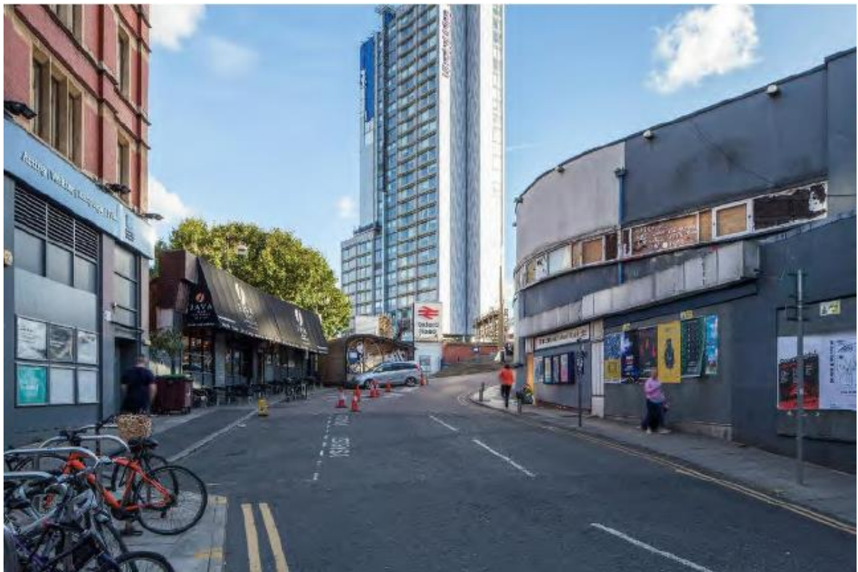
Viewpoint 6 – Oxford Road Station (existing)
