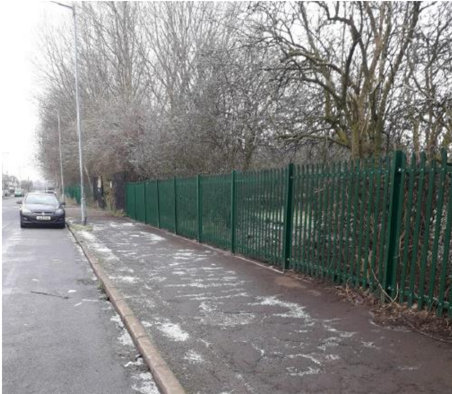
View along Cringle Road following completion of the works
