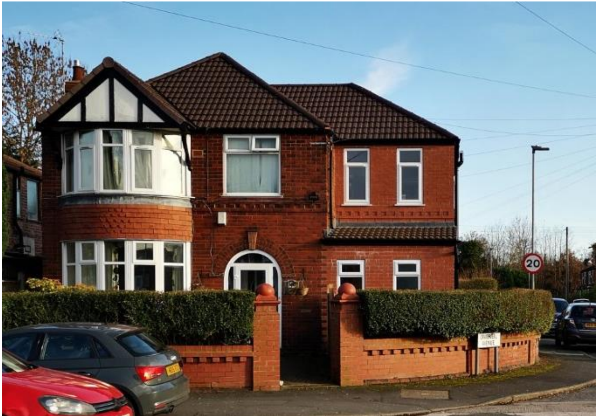
Number 367 Parrs Wood Road and completed site extension
