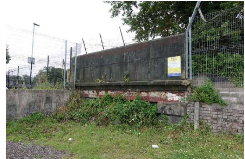
^ Existing bridge remnants of the old canal arm under Jersey Street
