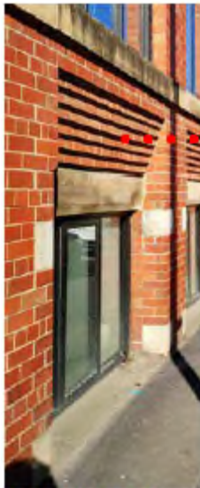
Brick detailing to openings - Britannia Mill
