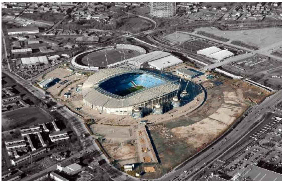
Figure one – existing stadium with the low slung roof at the south and north stands.
