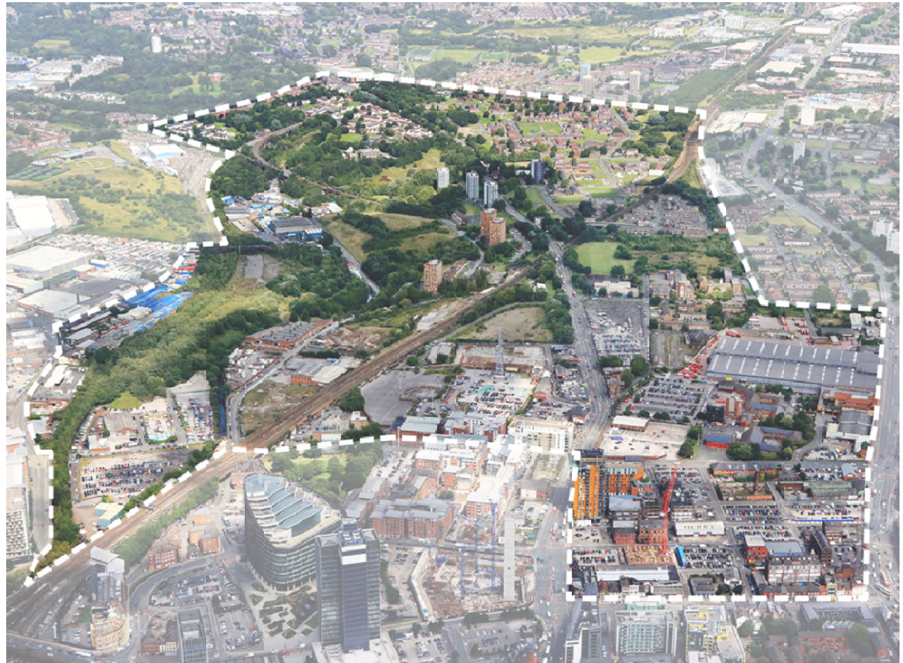
Figure 2 - Aerial view of the Northern Gateway
