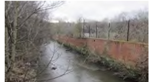
3. View of River Medlock looking South
