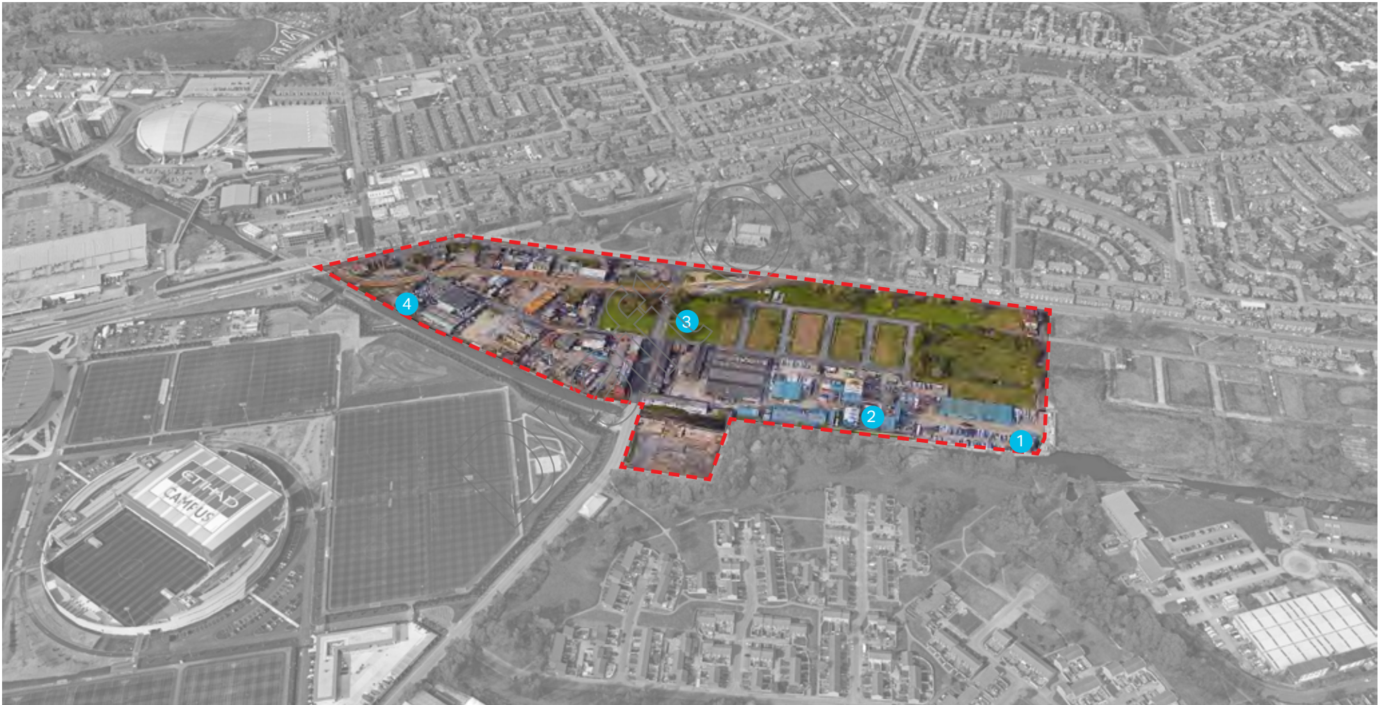
Figure 7.13 Aerial view of the regeneration area from south
