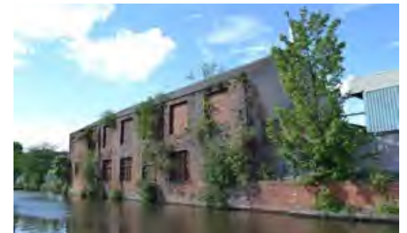
4. View of canal side warehouse
