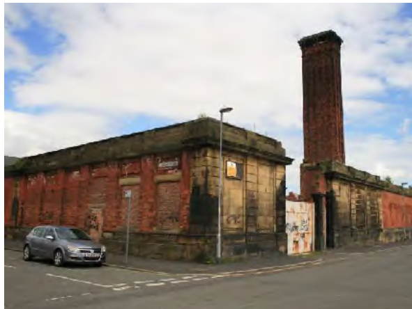
Highway lighting column
