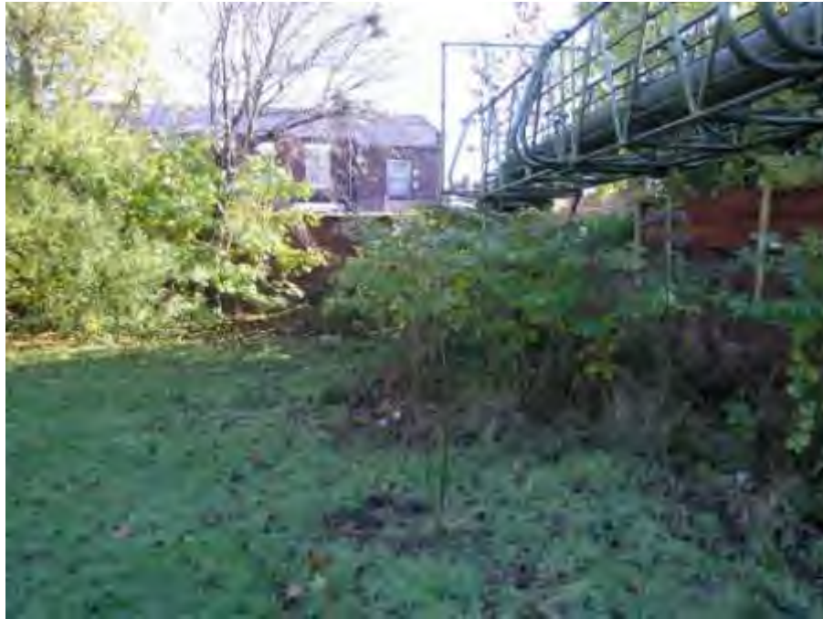
Photo 8 – Japanese knotweed under the elevated pipe
