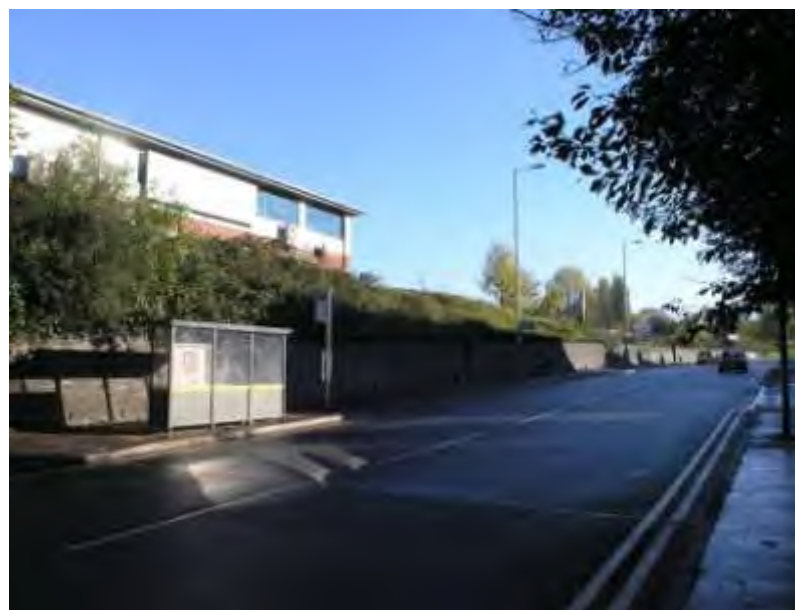
Photo 11 – Brick retaining Wall
