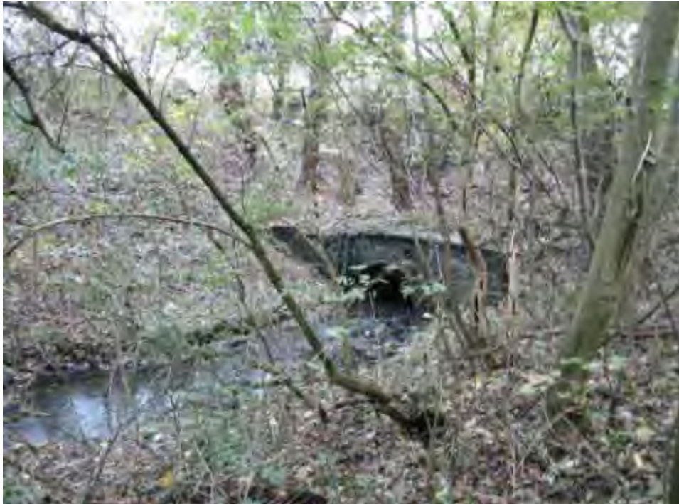
Photo 6 – Gore Brook culvert
