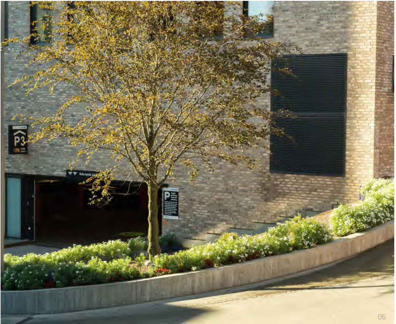
05 | Underground car parking
