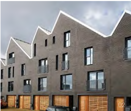
02 | Sustainable design that is solar efficient
