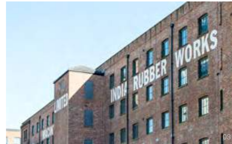
03 | Macintosh Mills, an early 19th century mills complex
