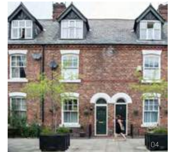
04 | Retaining the historic fine grain
