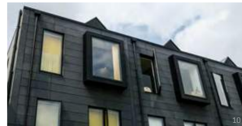
10 | Modular cost benefits houses, New Islington
