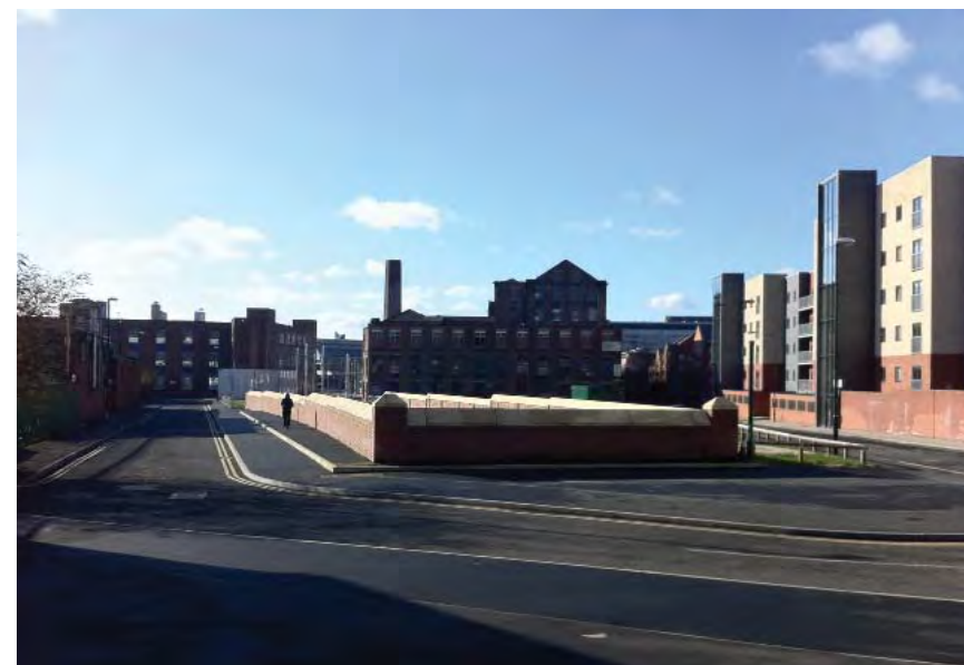
The Metrolink tunnel at Great Ancoats Street
