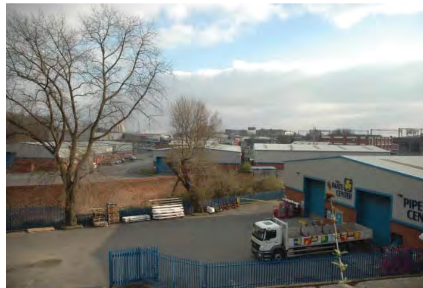
River Medlock concealed in an area of light industrial development
