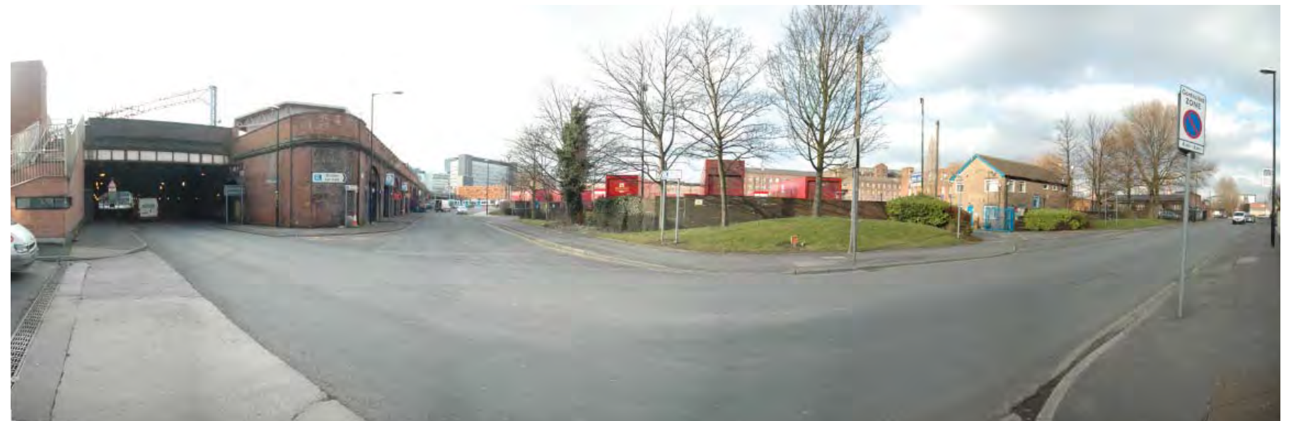
Existing rail viaducts and under developed land
