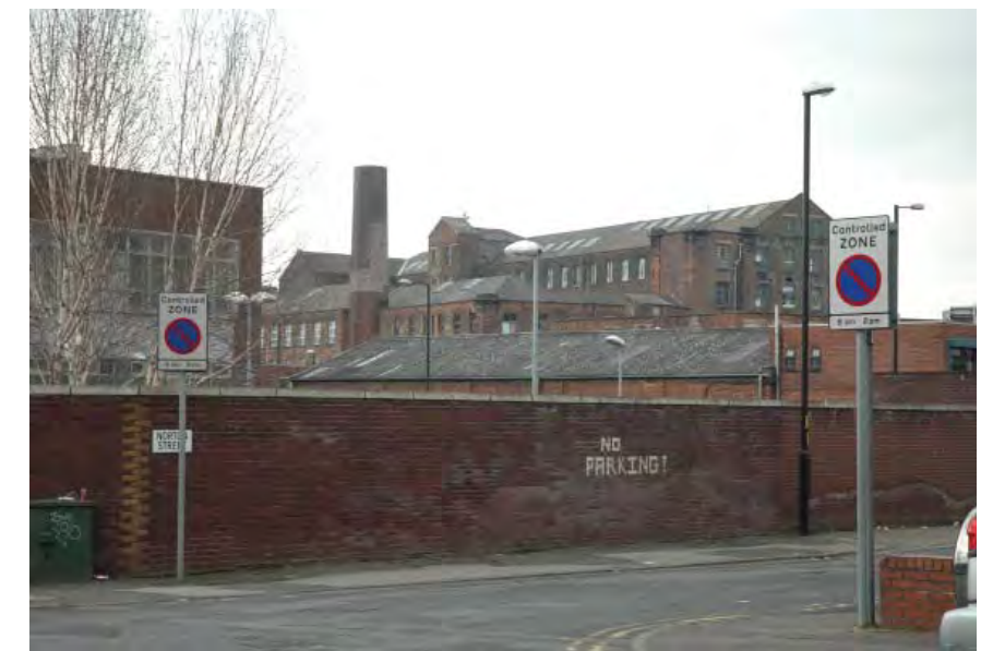
Existing mill buildings to be retained
