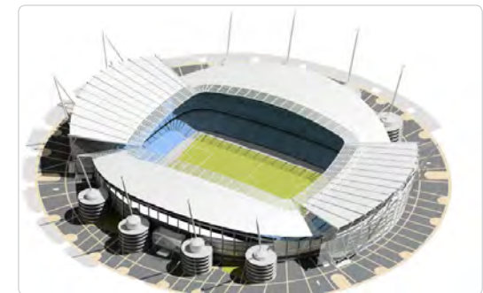
Expansion may occur at either, or both, the north and south ends
