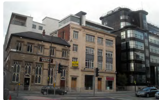
Upper portions of Great Ancoats Street have a more intact fabric
