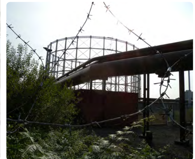
The Gasholder lands
