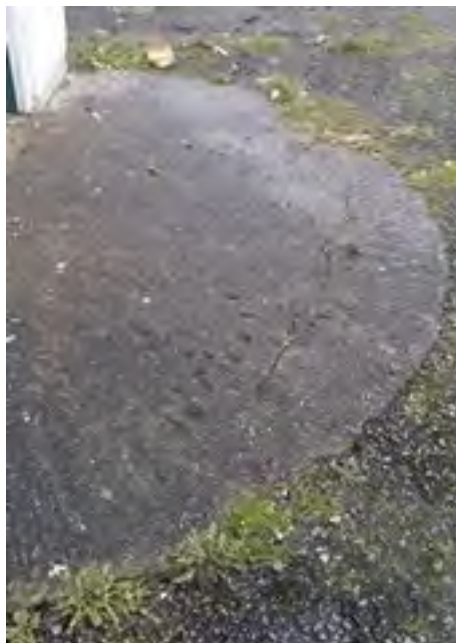
Ramped entrance to smaller room from car park.
