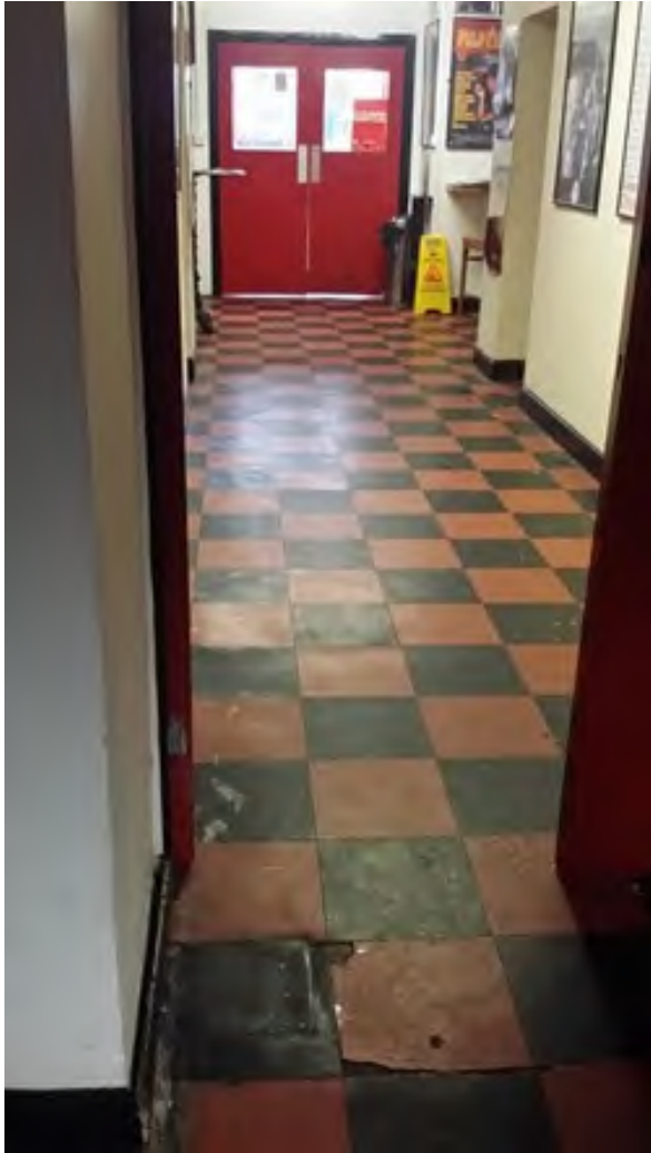
Corridor from main entrance to large room, with patterned floor and damage to floor
